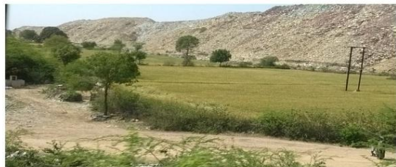
Deposits on Jhalwar-Ramganj Mandi highway
